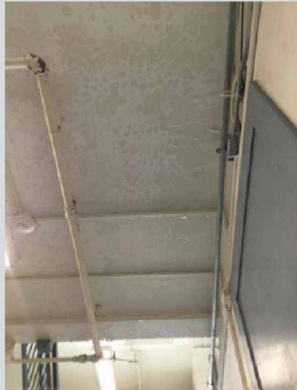
Ceiling & Wall Conditions
