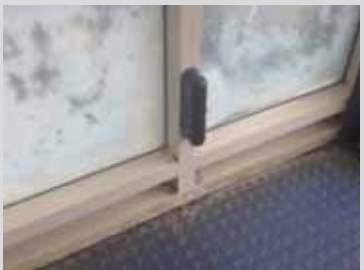
3. Motion sensors used to activate the sliding doors.
