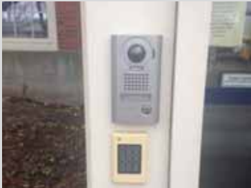
1. Video intercom and card reader at the door.
