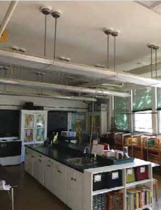
1938 Classroom Lighting: Pendant Mount Fluorescent Fixtures: Fair Condition
