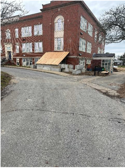
Outside view of the existing school
