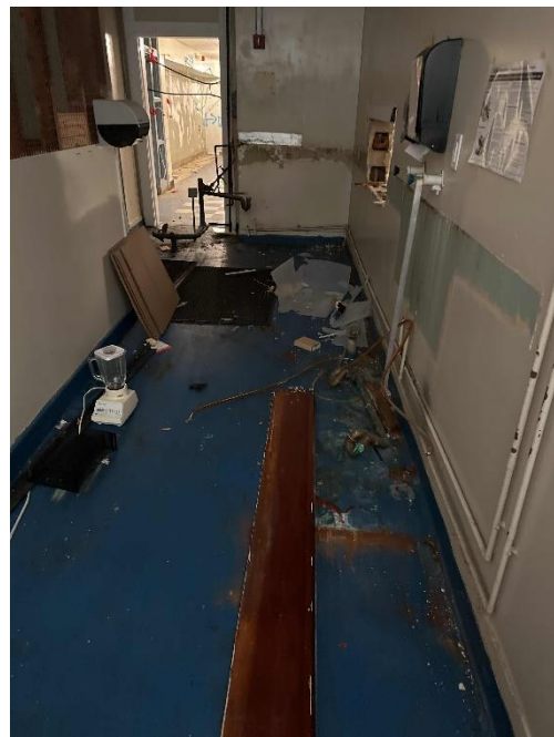
Abatement and selective demolition of existing building
