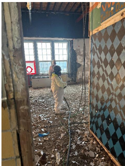
Abatement and selective demolition of existing building
