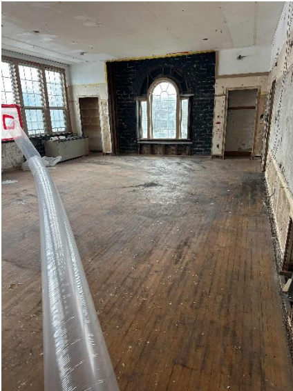
Abatement and selective demolition of existing building
