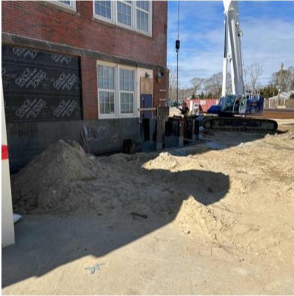
Secant Pile Installation
