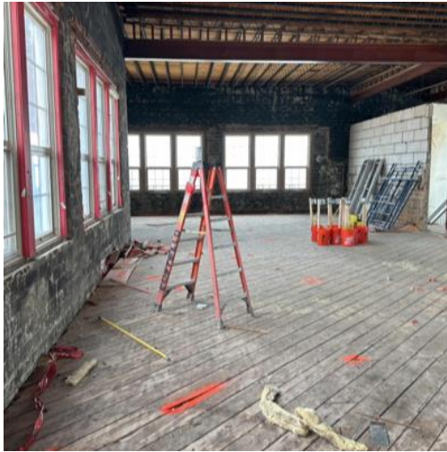
3 rd Floor Demolition Progress
