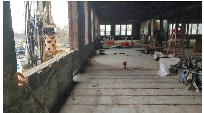
Window Removal 2 nd Floor
