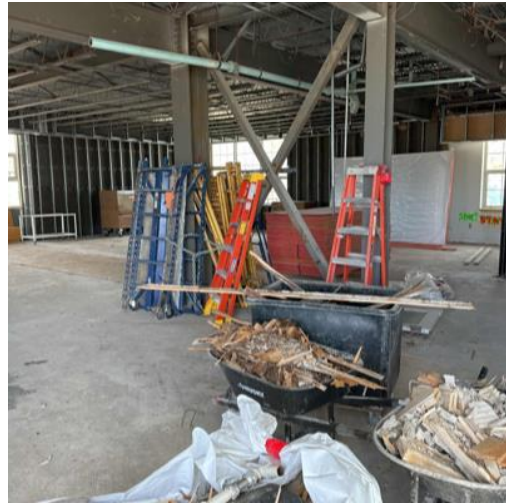
1 st Floor Demolition Progress
