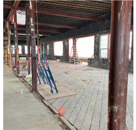
Temporary Window treatment
