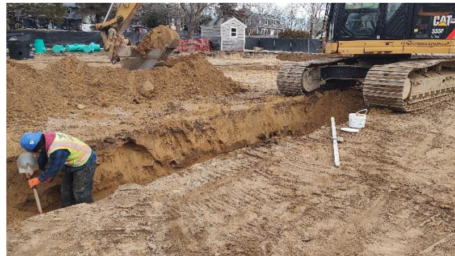
Excavating & Installing Drainage Pipe on West Side Playground Field Area
