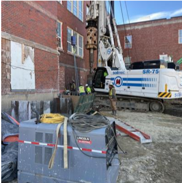
Secant Pile Installation
