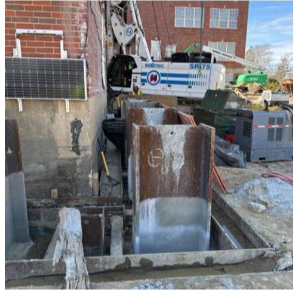
Secant Pile Installation
