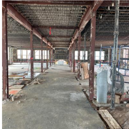
2 nd Floor Demolition Progress
