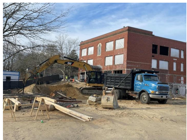
Cut at northeast corner of site
