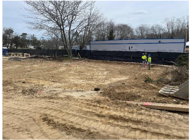
layout at east end of site
