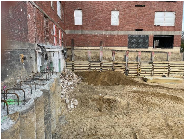
Finishing up work at pilings
