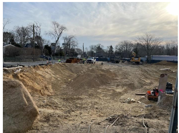
Trench along northside of site
